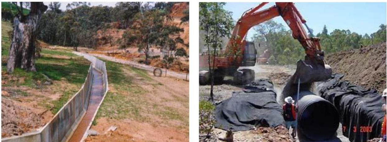
**Figure 108: Dawesley Creek diversion drain. Laying pipe for the underground segments of the drain (right) and open channels (left). Photos from Cox et al., 2006**
