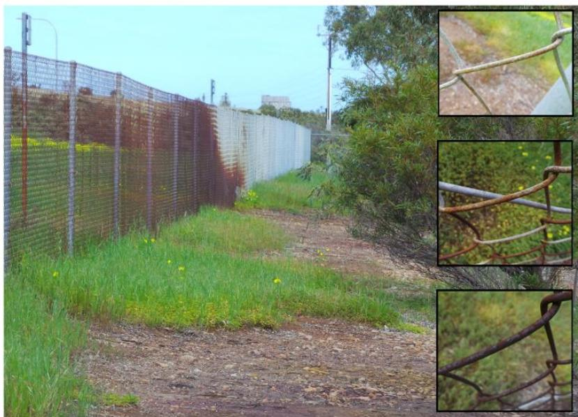
**Figure 44: Photographs showing the condition of fencing on Garden Island (South Australia). The section of the fence, which is heavily impacted by corrosion damage is located above Anthropogenic sulfuric silty soils, which originated from a sulfuric acid manufacturing plant.**
