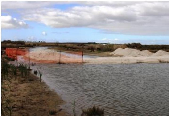
**Figure 19: Applications of fine limestone in the Finniss River below Wally's Landing jetty to acidic waters flowing from the wetland and channel in May 2009. (From Fitzpatrick et al. 2011d)**
