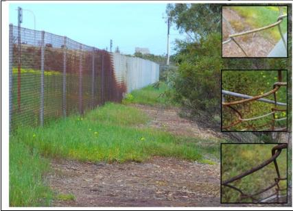
Fig. 1 Photographs showing the condition of fencing on Garden Island (South Australia). The section of the fence. is which heavily impacted by corrosion damage is located above Anthropogenic sulfuric silty soils, which originated from a sulfuric acid manufacturing plant.
